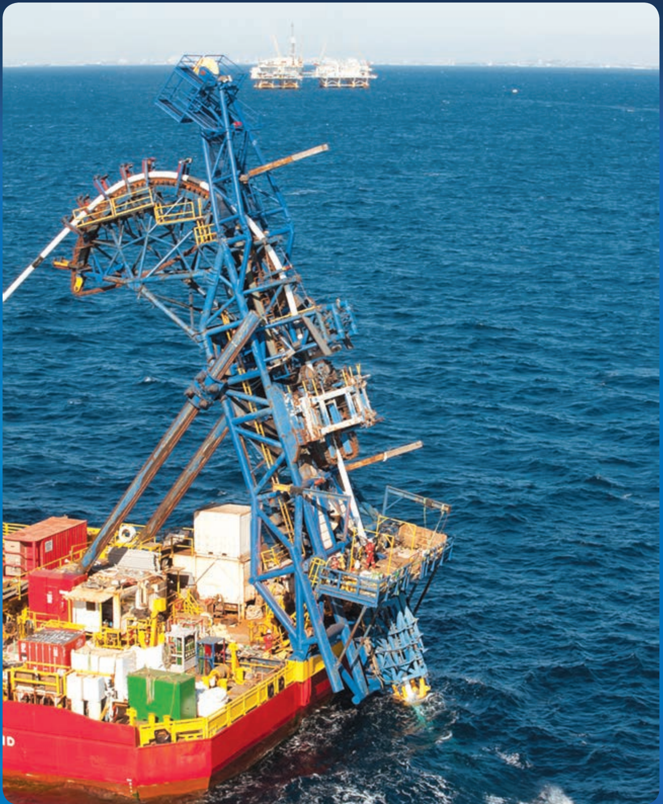
U. S. Steel Tubular Products seamless line pipe installation at the Helix Beta Offshore California project. Photo provided by Helix Energy Solutions Group.
