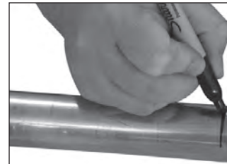
Figure 3 — Marking for Insertion Depth
