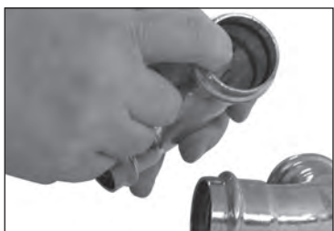
Figure 2 — Check for EPDM Seal
