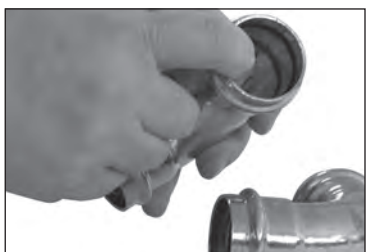
Figure 2 — Check for EPDM Seal
