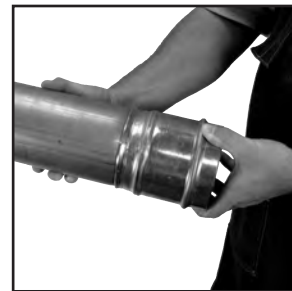
Figure 9: Inspection of final crimp
