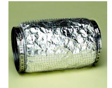
Clamp second end of ArmorMesh to liner and trim excess ArmorMesh.
