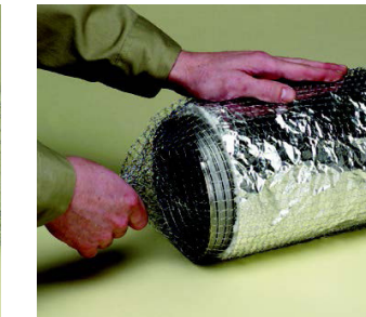
With one end of ArmorMesh clamped to the liner, pull the other end to snug along entire length.
