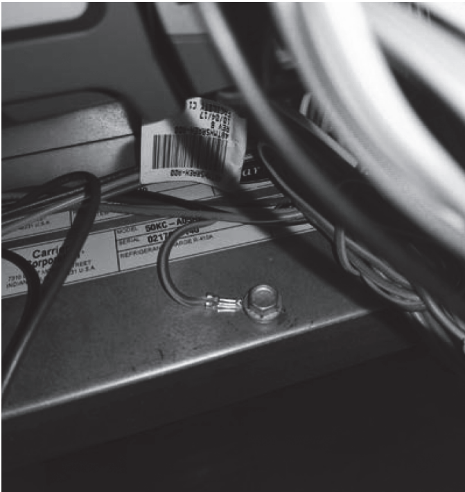
Fig. 12 — Connect Ground Wire From Controller
