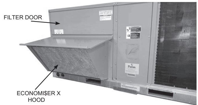
Fig. 20 — Install EconoMi$er X Hood and Unit Filter Access Door
