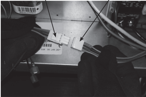
Fig. 13 — Connect 48TMHSRSE--A20 Harness to Harness from Controller
