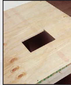
Cut the hole.
