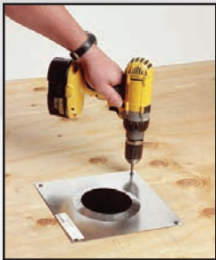
Mount SureGrip support plate.
