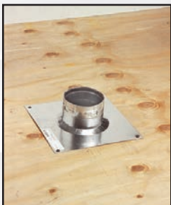
Push pipe through vent support.
