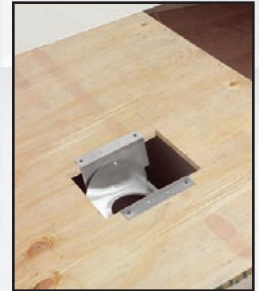
Mount SureGrip support plate.
